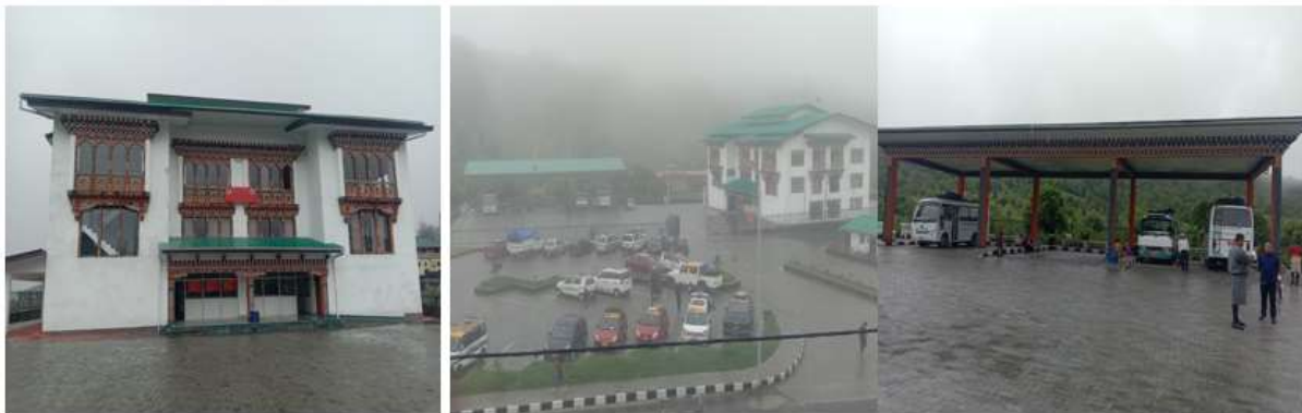
Tsirang Base Office
