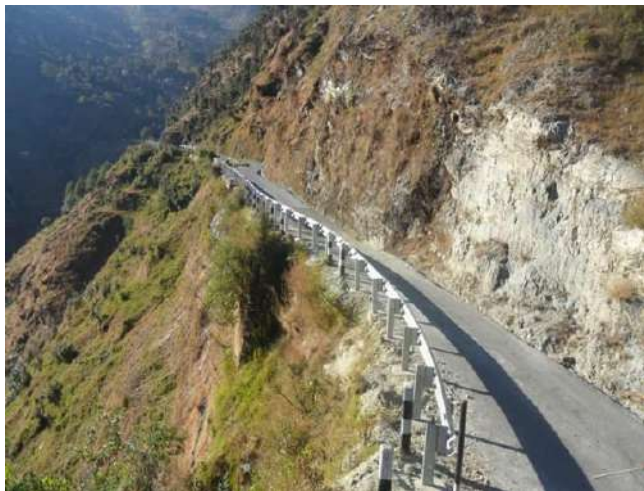
Figure 4.4: Roadside Barriers in Nepal. The GRSF funded construction of roadside barriers on cliff-side roads in Nepal, showing in order the road without barriers, during construction, at completion, as well as an example of a bus which was prevented from going over the cliff by the barrier
