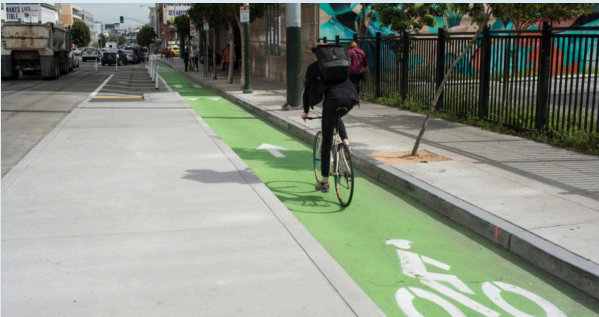
8th Street in San Francisco after being treated with a protected bike lane coupled with a passenger loading island. Source: SFMTA
